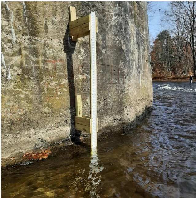
Figure 2. Staff gage installed at the Salmon River Trestle Pool project site.
